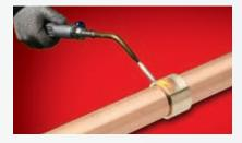
If the complete ring of solder does not appear on heating, apply additional flux to the mouth of the socket and end feed the joint with our N165 (Copper coloured) or N166 (Brass coloured) cadmium-free silver brazing alloy, or an equivalent to the compositional requirements of BS EN 1044 AG103 (formerly BS 1845 AG14).
